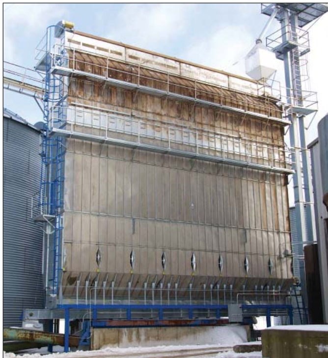
New Delux Mfg. DPX 3,280 bph tower dryer at Door County Cooperative's Shirley Feed Mill in De Pere, WI.
