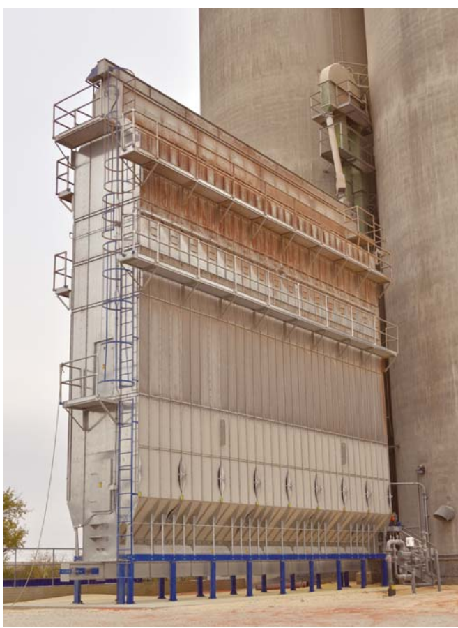
New Delux DPX16GT Series dryer at FC Cooperative's elevator in Afton, IA is rated to remove five points of moisture at 3,200 to 3,500 bph depending on the commodity. Photos by Ed Zdrojewski.
